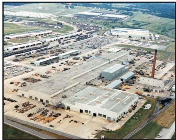
An ariel view of the completed buildings 350, 370 and 320 are ready for the new Paladin mission as well as other tracked, wheeled vehicles and the new missile workload.
